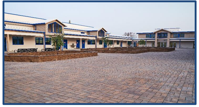
Sunset High School / Campus Re-construction
