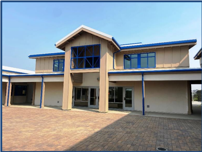
Sunset High School / Campus Re-construction
